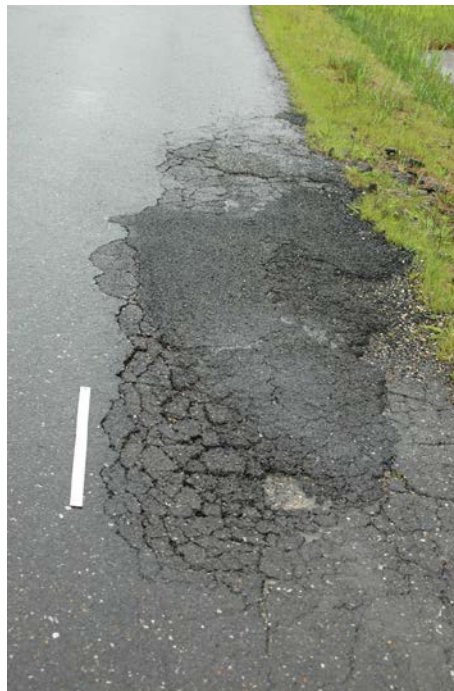
Typical Paved Road Deterioration
