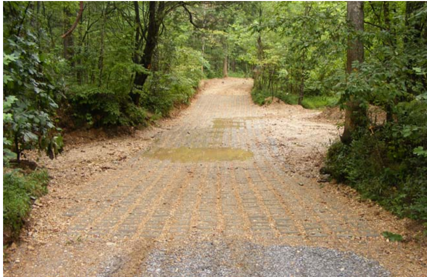
Hardened stream crossing in Turkey Bay OHV Area.
