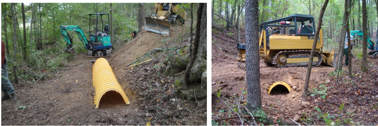
Figure 7.4. Installation of open bottom arch culverts
