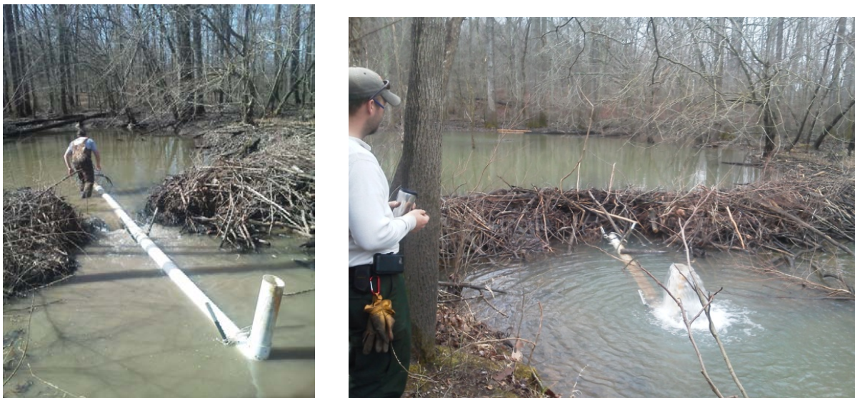
Figure 7.6. Pond leveler installation at beaver dam.
