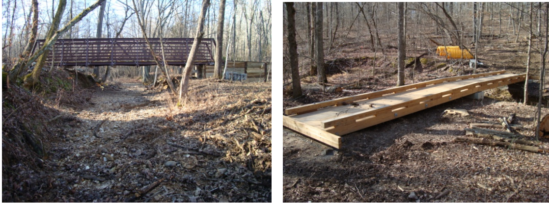
Figure 7.3. Installation of trail bridges.
