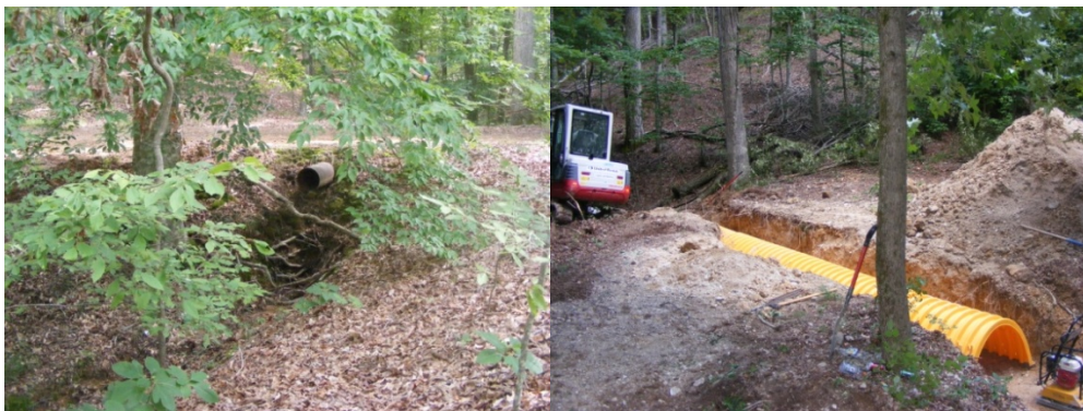
Figure 7.7 Wrangler's Trail #1 Culvert Replacement
