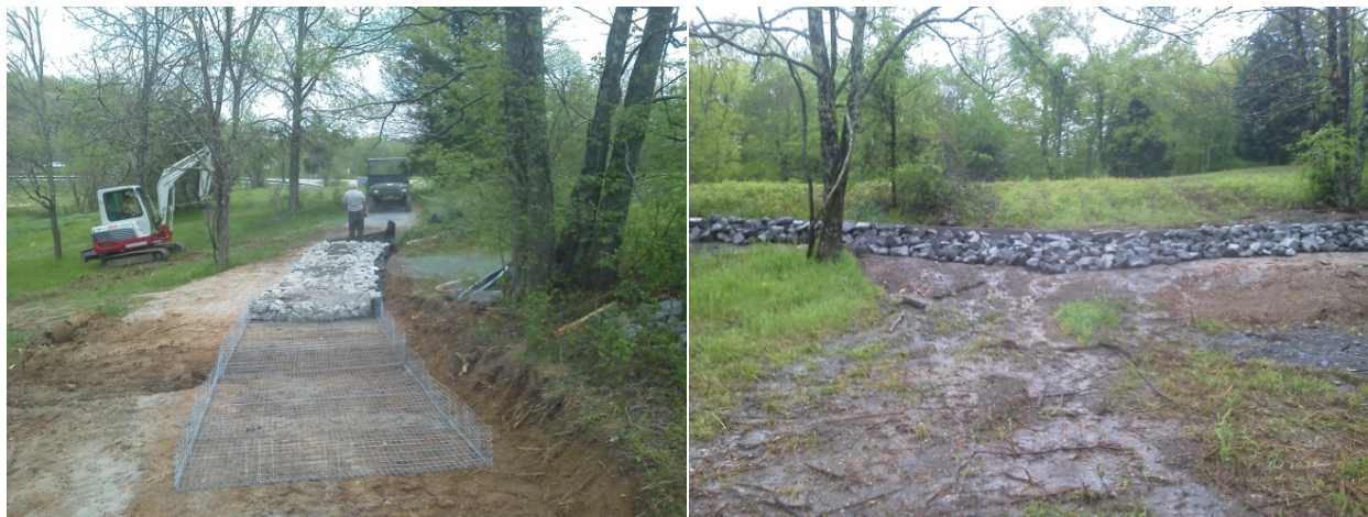
Figure 7.8 Central Hardwoods Scenic Trail gabion mattresses
