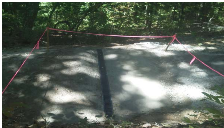
Figure 7.9 Central Hardwoods Scenic Trail trench drain
