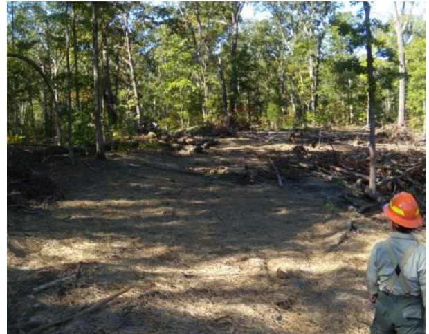
Figure 31: We used seed, mulch, and timber slash on a skid trail in the Jenny Ridge timber sale to mitigate soil erosion and water run off
