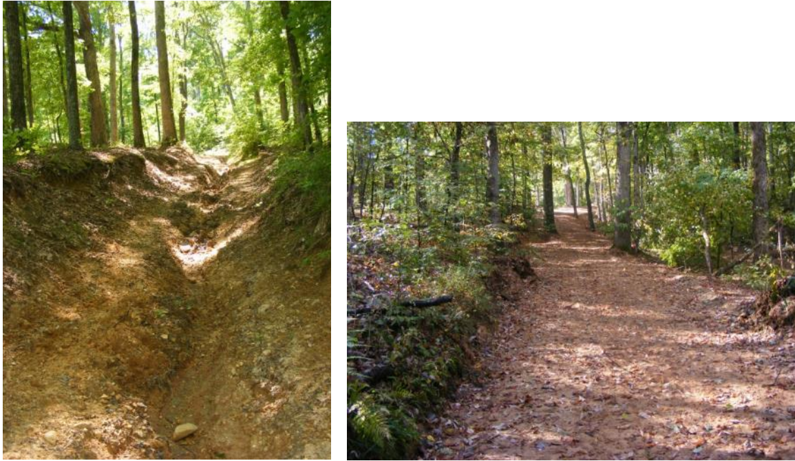
Figure 52: We filled the entrenched Wranglers Trail #4 and installed appropriate water drainage structures using onsite material as can be seen in these before and after photos
