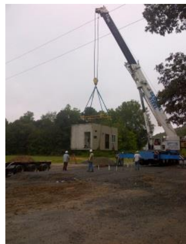
Figure 48: Installing the precast gatehouse at Turkey Bay OHV Area in early FY2015
