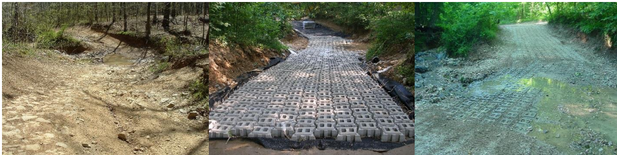
Figure 7.20: One of eight creek crossing stabilization projects in Turkey Bay OHV Area (before, during, after)
