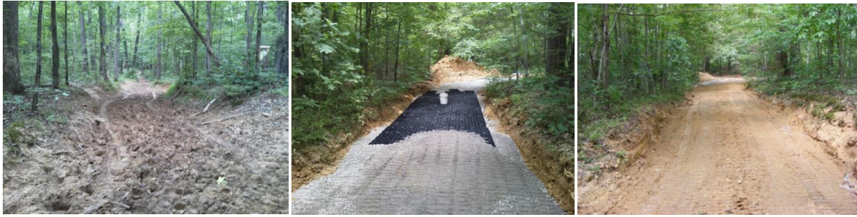
Figure 7.7: Repairing a poorly drained section of Wranglers Trail 6, 1997/98
