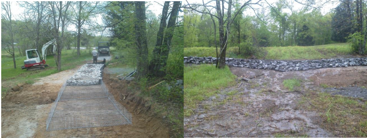
Figure 7.7: Repairing a poorly drained section of the Central Hardwoods Scenic Trail
