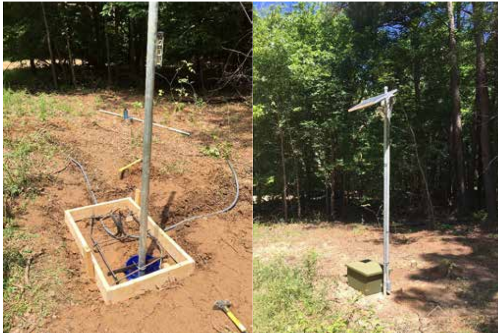
Figure 7.28: New soil moisture monitoring station at Turkey Bay Off-Highway Vehicle Area (June 2017)
