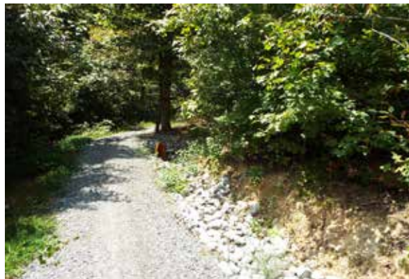
Figure 4.2: BMP of rock armored ditch and culvert on the Central Hardwoods Scenic Trail
