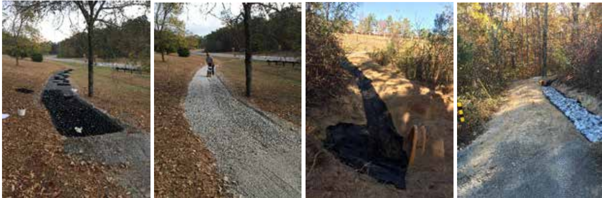
Figure 7.26: Repairs to poorly drained sections of the Central Hardwoods Scenic Trail (October-November, 2016)
