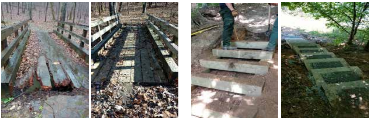
Figure 7.27: (Left) North/South Trail bridge decking repairs (May-June, 2017); (Right) Honker Trail steps replacement (June-July, 2017)
